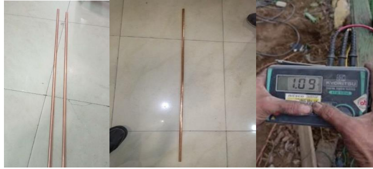
Fig. 4. Repair results and addition of electrodes on the Alarm panel
