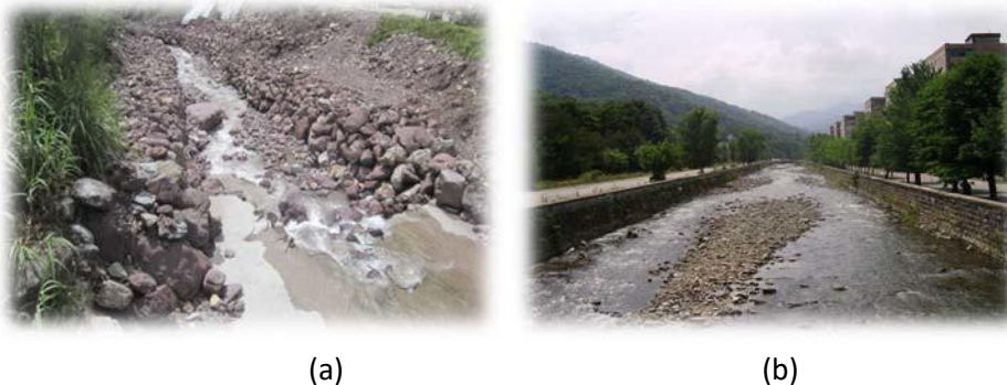
Figure 13. (a) Normalization using natural rocks, (b) Normalization using vertical gabions (source: https://estuarymetal.com/normalization-vs-naturalization )
