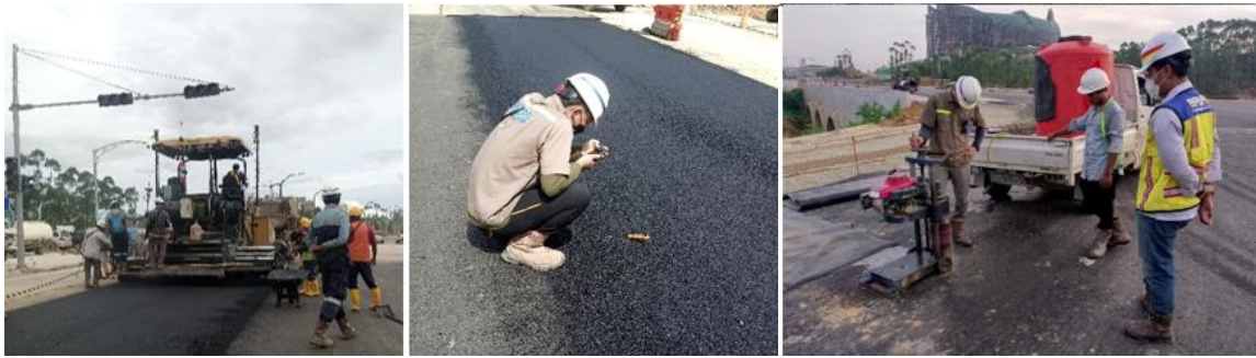
Gambar 3. (a) Proses pengaspalan; (b) Pengambilan Sampel Core Drill
