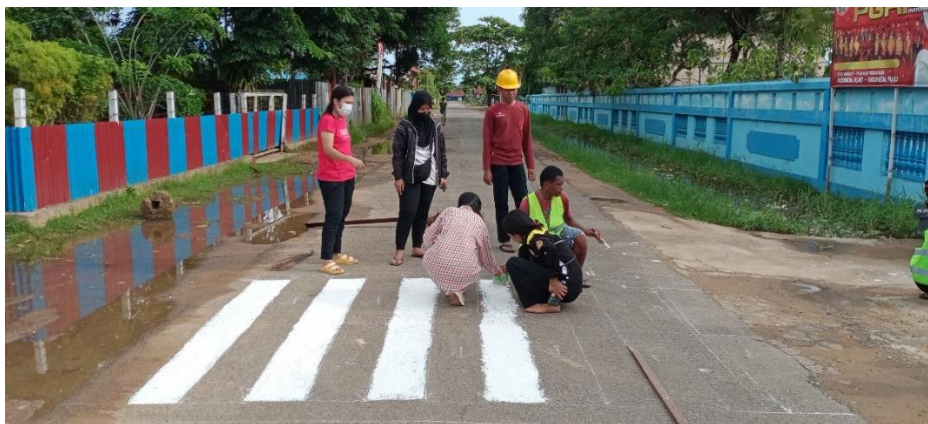
Gambar 8 Proses pengecatan Zebracross
