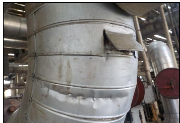
Figure 6. Window Opening for CUI Inspection
